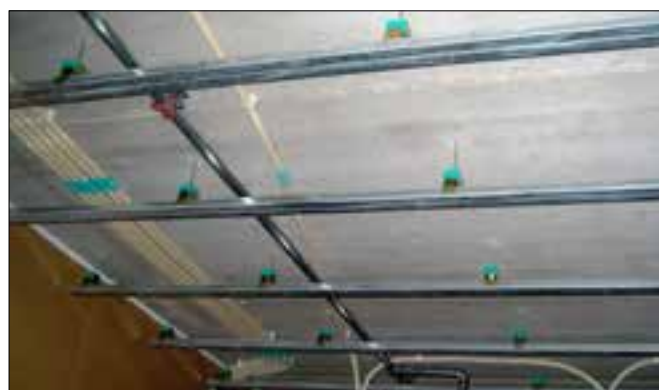
Application of an Akustik Super T60 +Sylomer 30 type B.
