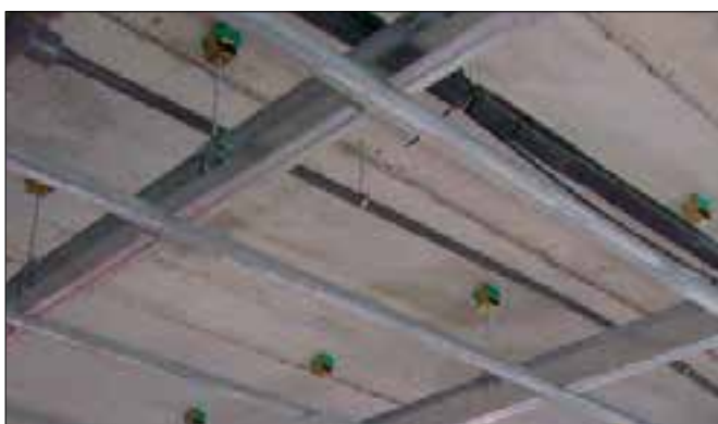
Application of an Akustik 4+Sylomer 30 type A.
