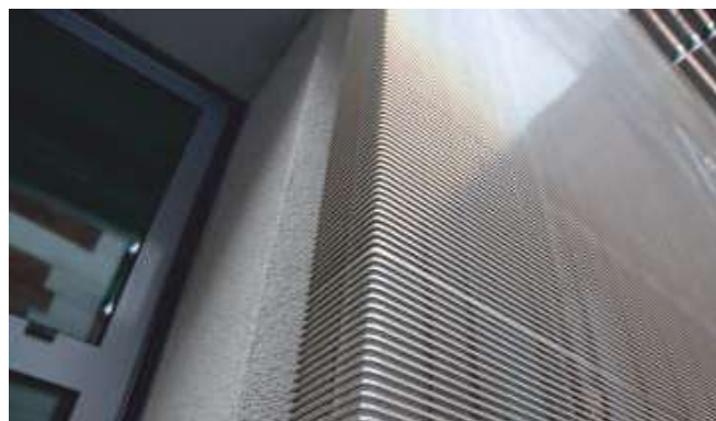
Facade grid bent in the vertical plane
