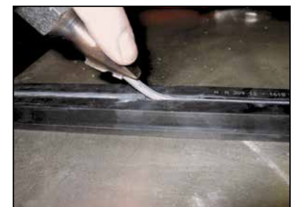
Installation of Datwyler Black Swell into the composite Tunnel gasket
